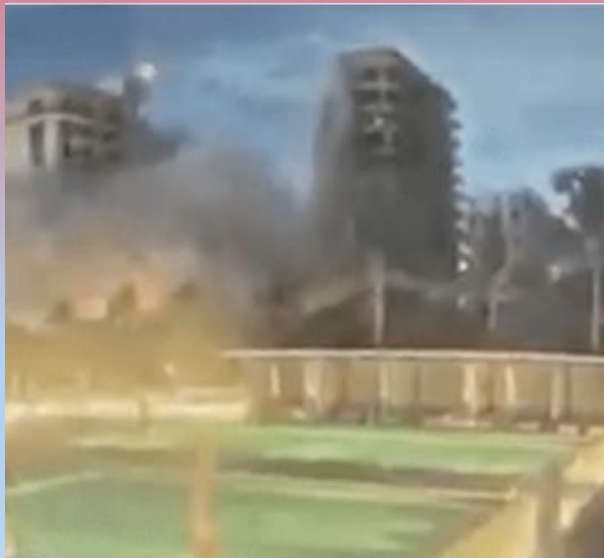
4 seconds Central section fully collapses
