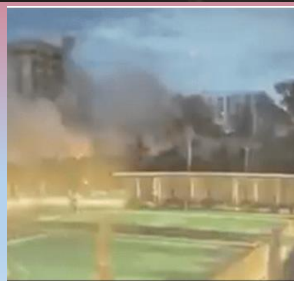
12 seconds East section fully collapses
